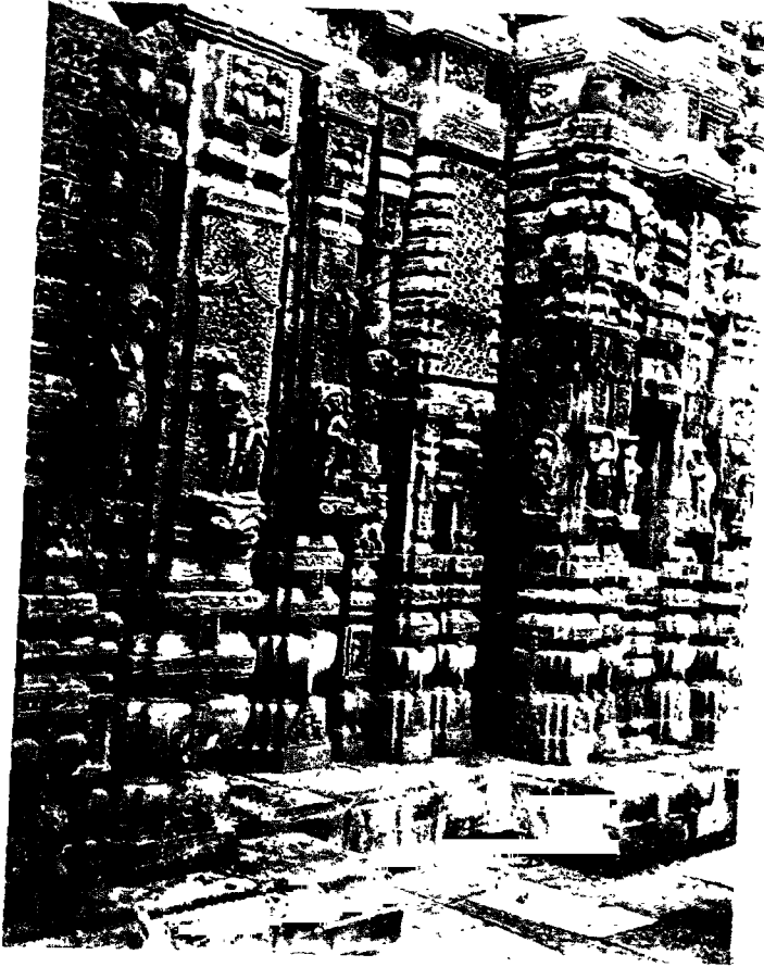
Facade of Muktesvara showing the plinth, pedestal and pilasters.
